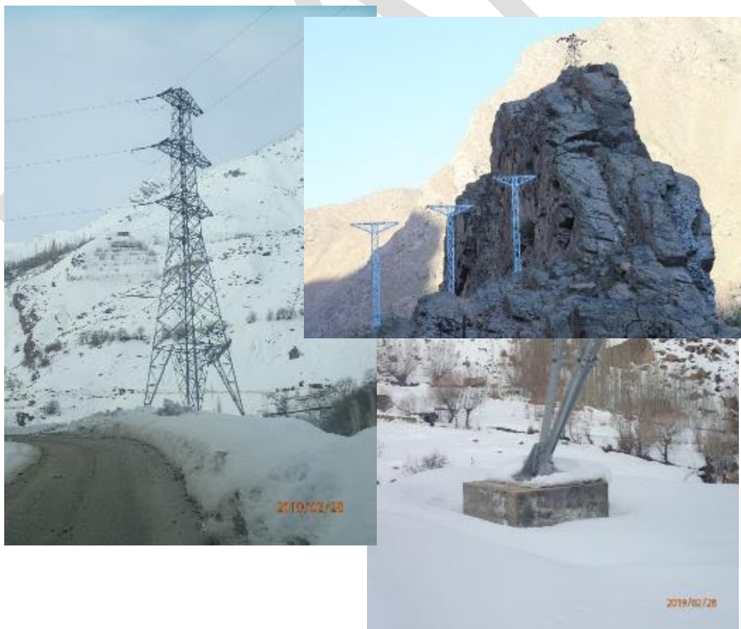
Figure 5. Examples of towers: angle tower at left, three suspension poles on uneven terrain at top right, example of foundation at lower right
